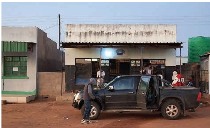
Businessmen at Tshitulipasi Business Centre enjoying electricity from the 120kW solar plant installed by REA late last year.
