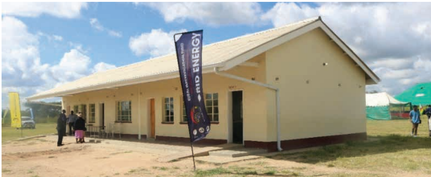
St Anna Mere primary school in Svosve Communal area, Marondera District in Mashonaland East province is one of many schools electrified by REA as from July last year.
