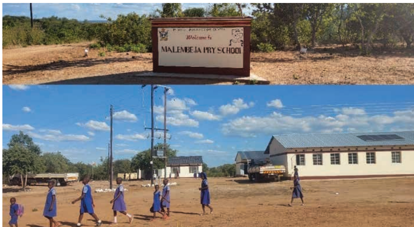
Newly electrified Malembeja primary school in Kariba district, Mashonaland West province
