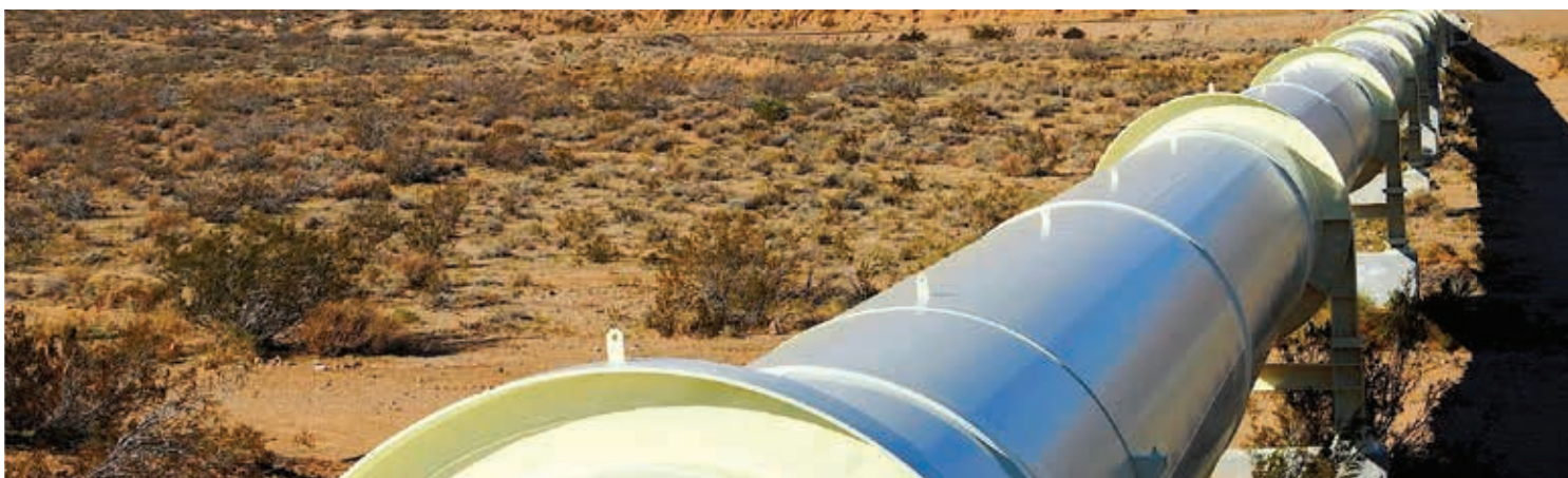
Beira-Feruka fuel pipeline capacity upgrade
