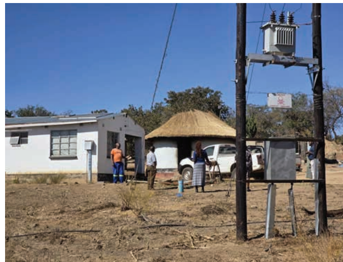
Chief Nhema's newly electrified homestead Shurugwi district, Midlands Province.
