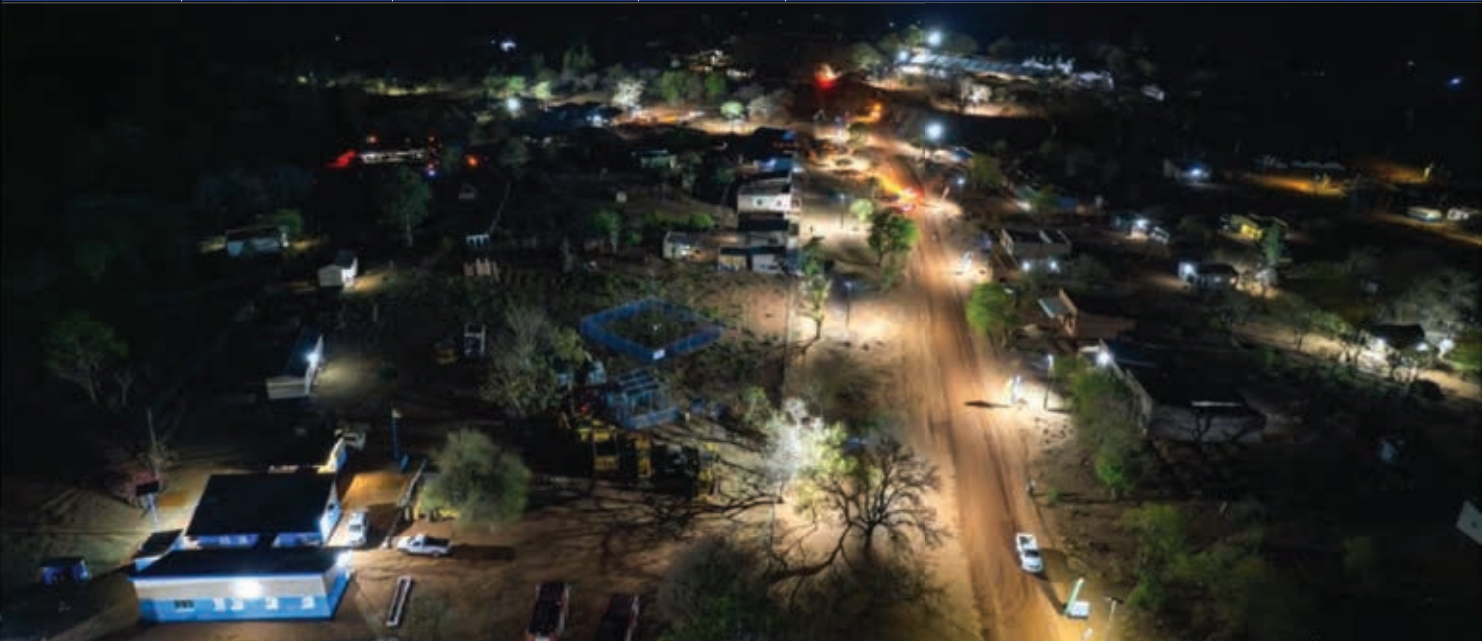
The Hwakwata Village Solar Mini-Grid Project.
